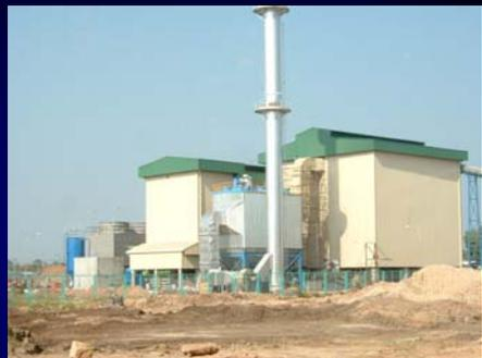
Uses rice husks, which are a by-product of the rice mill, to generate electricity as well as to reduce the volume of waste
