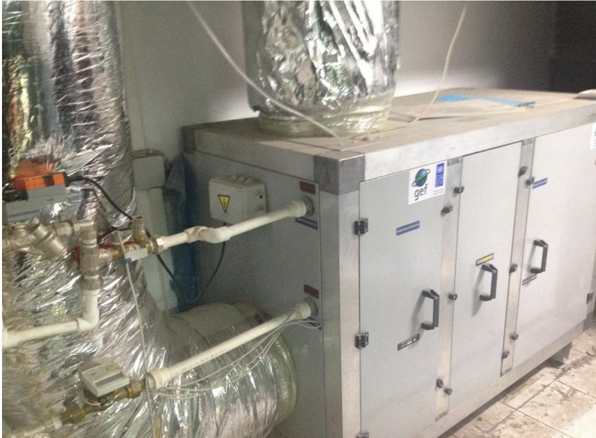
Energy Efficient Buildings in Kazakhstan 2015 GEF 3758
