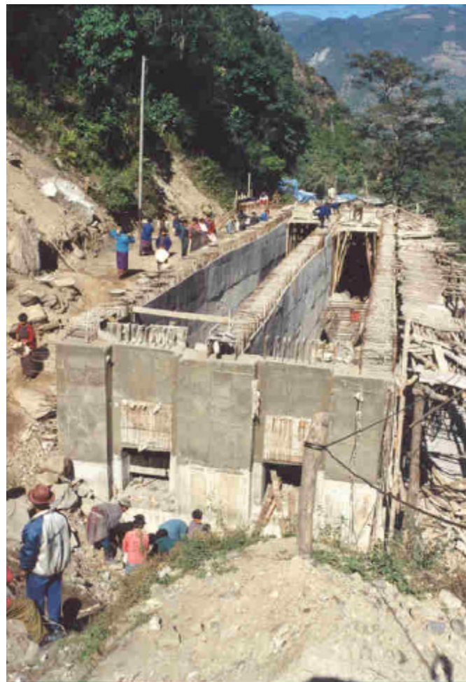
Figure 32: The double-basin sand trap under construction in December 2000
