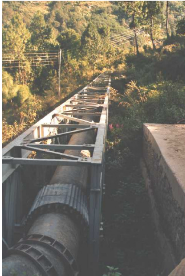
Figure 46: Pipe bridge crossing the potentially unstable slope on the Rangjung headrace
