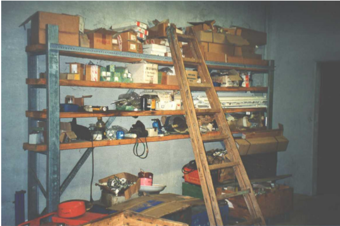
Figure 48: Electrical spare-part store at the Rangjung powerhouse
